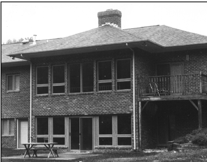
This North Carolina home uses a sunspace with a properly sized overhang. The sunspace can be isolated from the rest of the house to protect living spaces from temperature extremes.
