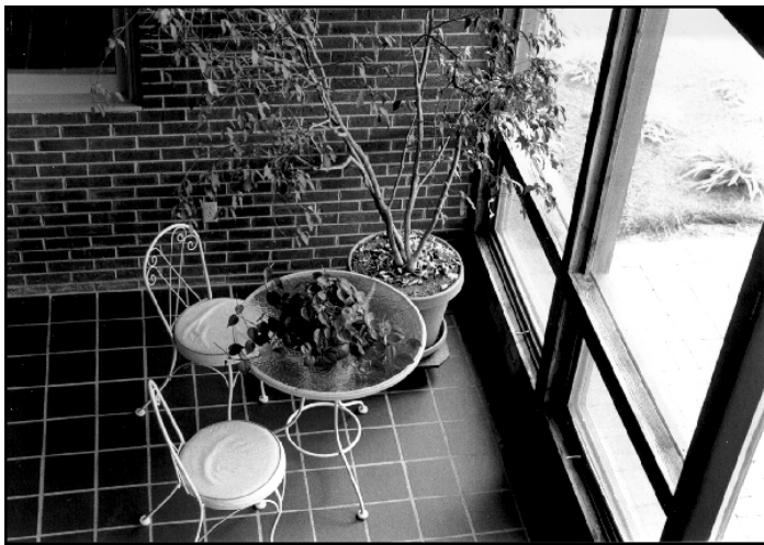
Tile floors and masonry walls provide thermal mass to store solar heat. Doors between sunspaces and other living areas can be opened to allow warm air to circulate.
