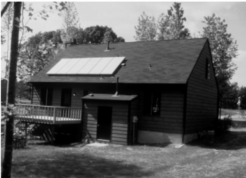
Fig. 11: Active solar space heating system.
