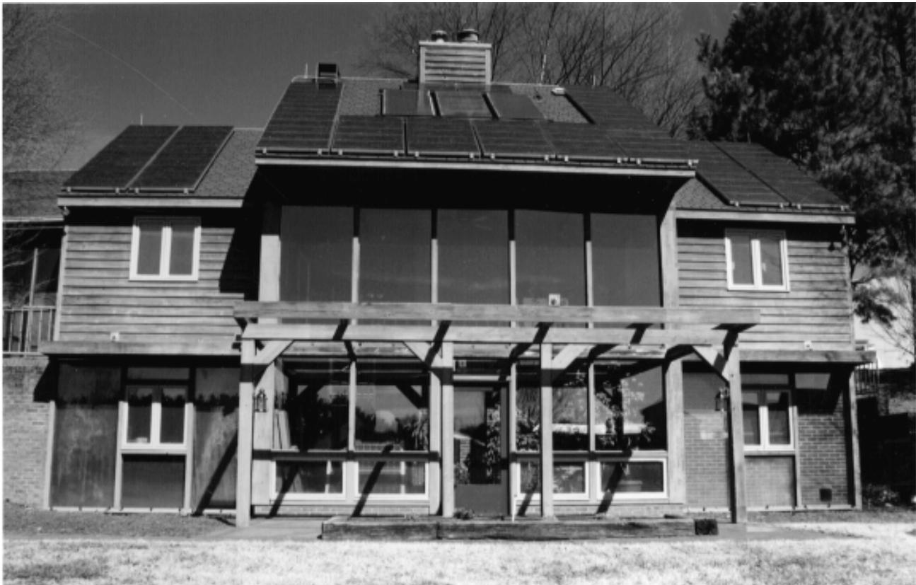
Fig. 3: The NCSU Solar House with direct gain, trombe walls, sunspace, active solar water heating system and photovoltaic electrical system.
