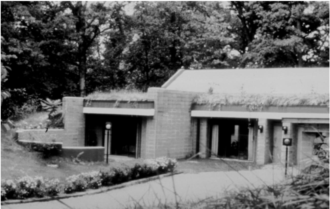
Fig. 16: Earth-bermed passive solar house.
